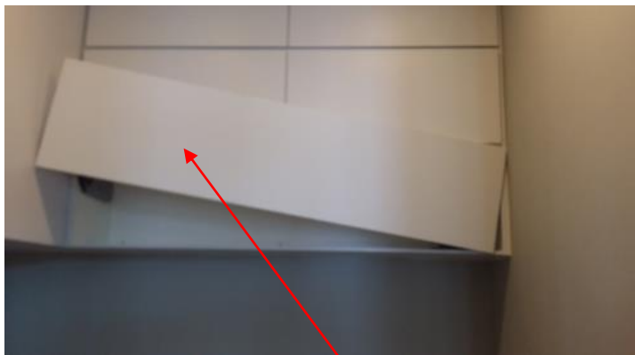
AVENTOS HL does not open properly.
